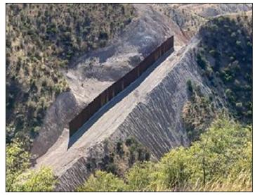
Erosion below the site of a cleared staging area (left); erosion below an area where only several border barrier panels were installed as of January 2021 (right).
