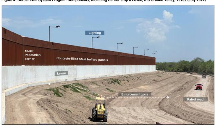
Figure 4: Border Wall System Program Components, Including Barrier atop a Levee, Rio Grande Valley, Texas (July 2022)
